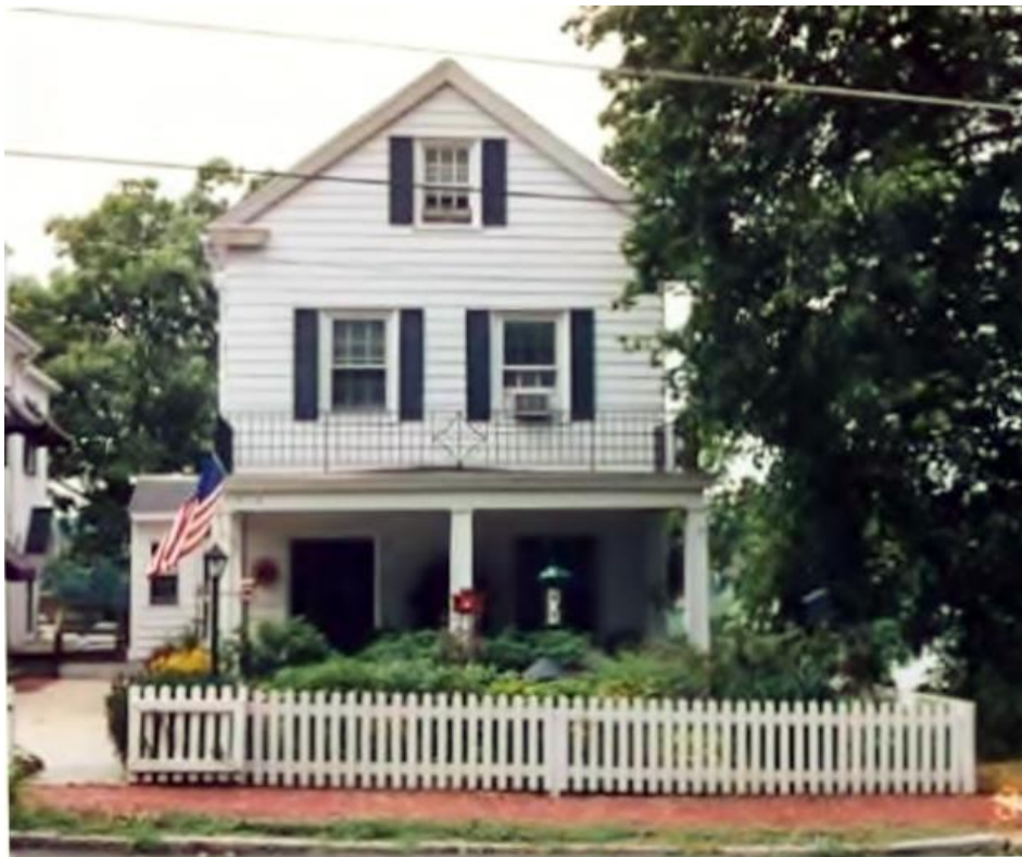
Parish Rectory at 1318 Howard Ave., Pottsville, PA
